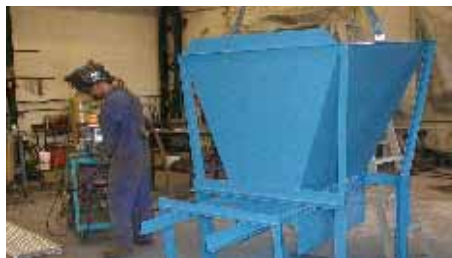
Fabrication of Equipment
