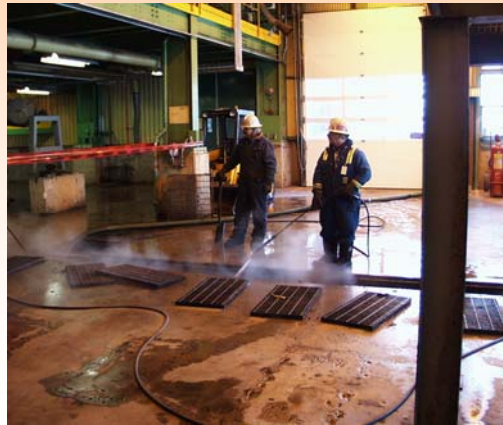
Leased space being cleaned out in preparation for construction activities (January, 2004).
